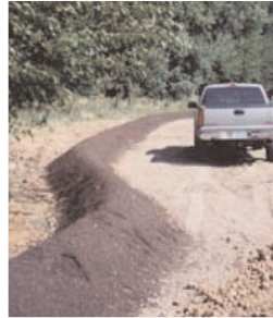
Compost Filter Berm
